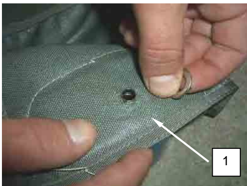
Figure 1. Insert Barrel of Replacement Grommet through Accommodating Hole.
