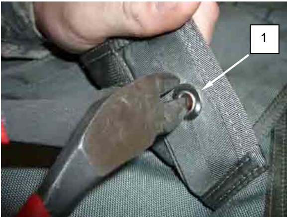
Figure 1. Remove Original Grommet.
