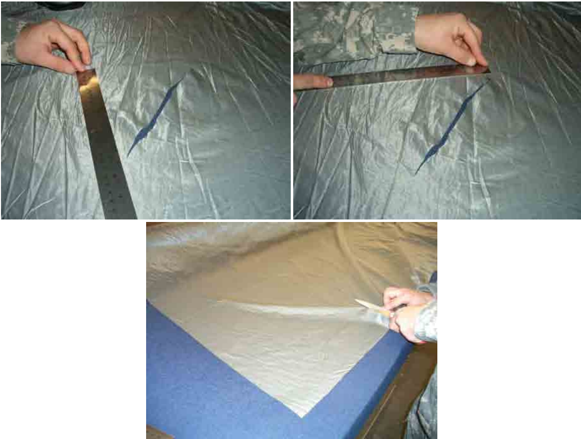
Figure 9. Measuring Damaged Area and Cutting Section of New Material.
