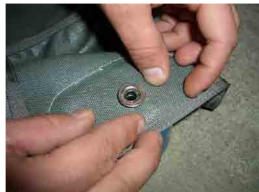
Figure 1. Insert Barrel of Replacement Grommet through Accommodating Hole.
