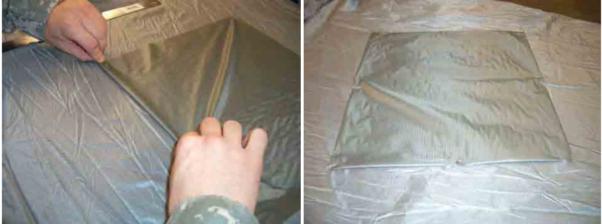
Figure 10. Placing New Material over Damaged Area and Securing with T-pins.
