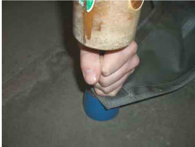
Figure 6. Spread Grommet Barrel.
