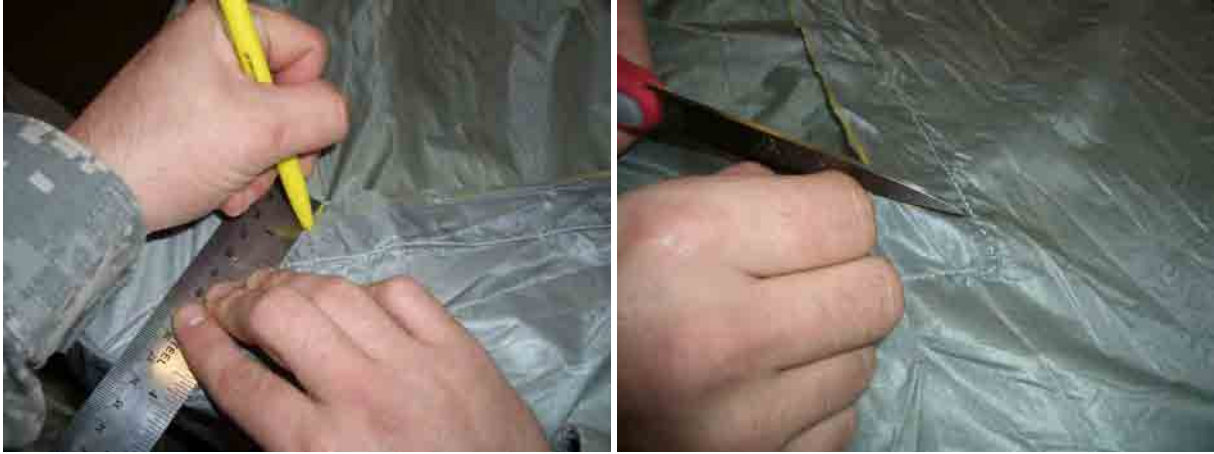
Figure 14. Cutting Patch Corners.
