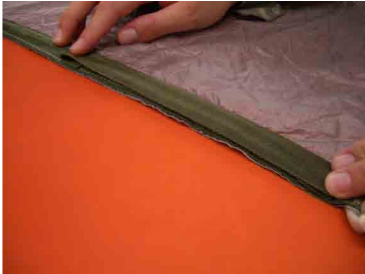
Figure 3. Place New Material Centered over Damaged Area.
